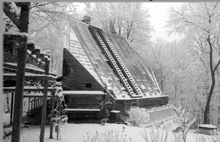
Figure 11.4: South face of the Raven Run Solar House. The permanent yet moveable ladder system allows for easy window maintenance and also provides shading during the summer months, Dick Levine
