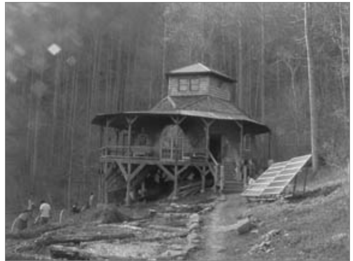
Figure 3.3: This off-the-grid home in Rockcastle County, Kentucky is powered by the PV array in front of the house, Andy McDonald
