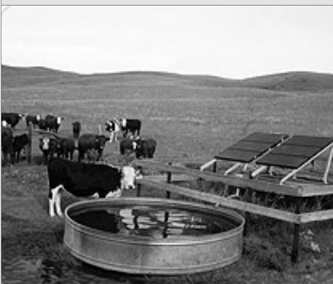
Figure 3.6: PV-powered water pumps provide water for livestock.
