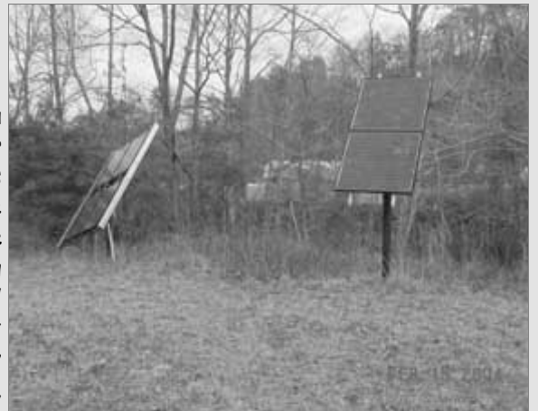
Figure 3.8: The tracking array shown on the left follows the sun throughout the day, increasing power output, Andy McDonald
