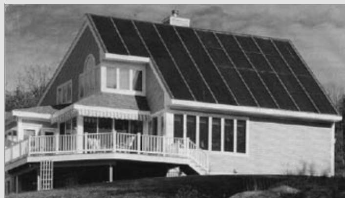
Figure 3.7: Building Integrated Photovoltaics (BIPV) can replace roofing shingles, as in this home.
