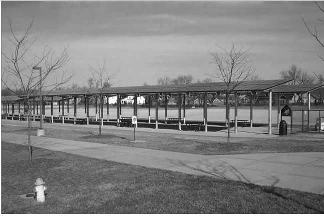
Figure 3.11: PV panels double as roofing for this pavilion at the Lover's Lane soccer complex in Bowling Green, Kentucky, Tennessee Valley Authority
