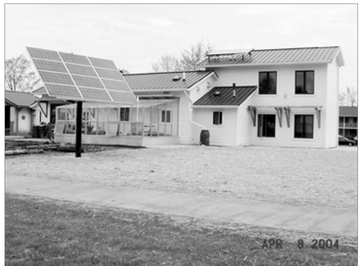
Figure 4.6: A tracking PV array at Berea College's Eco-Village Andy McDonald
