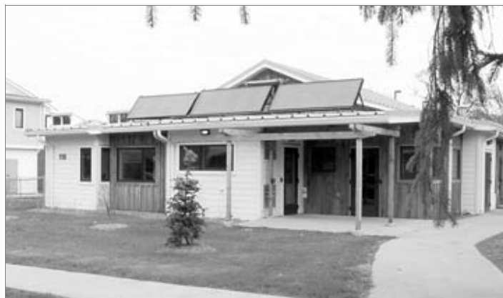
Figure 7.7: Solar water heater at Berea College. Andy McDonald
