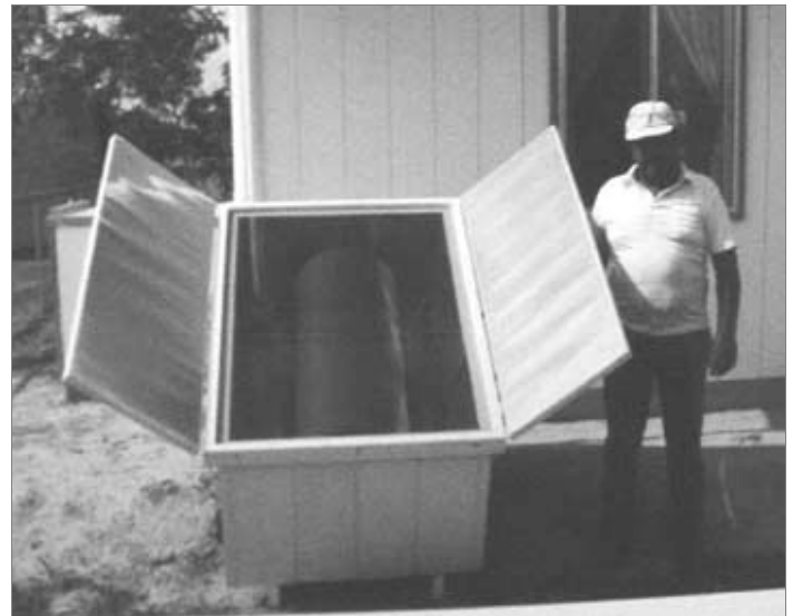
Figure 7.2: This batch solar water heater in South Texas provides year-round hot water, David Omick
