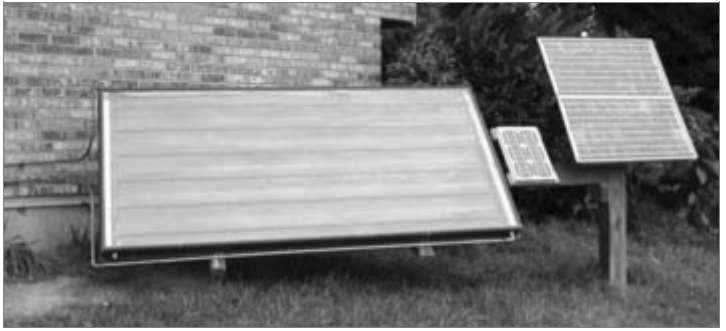
Figure 8.6: This flat plate solar collector (left) is mounted on the ground outside a home in northern Kentucky. This glycol antifreeze system uses a small PV panel (center) to pump the antifreeze through the system, John Robbins
