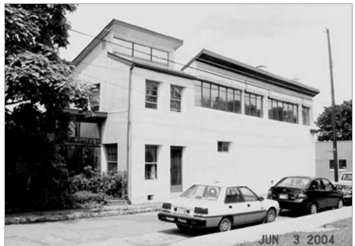
Figure 8.2: This home in Louisville has a batch solar water heater located inside the living space, which provides freeze protection and allows for year-round use. The water heater is located behind the high windows on the left.
